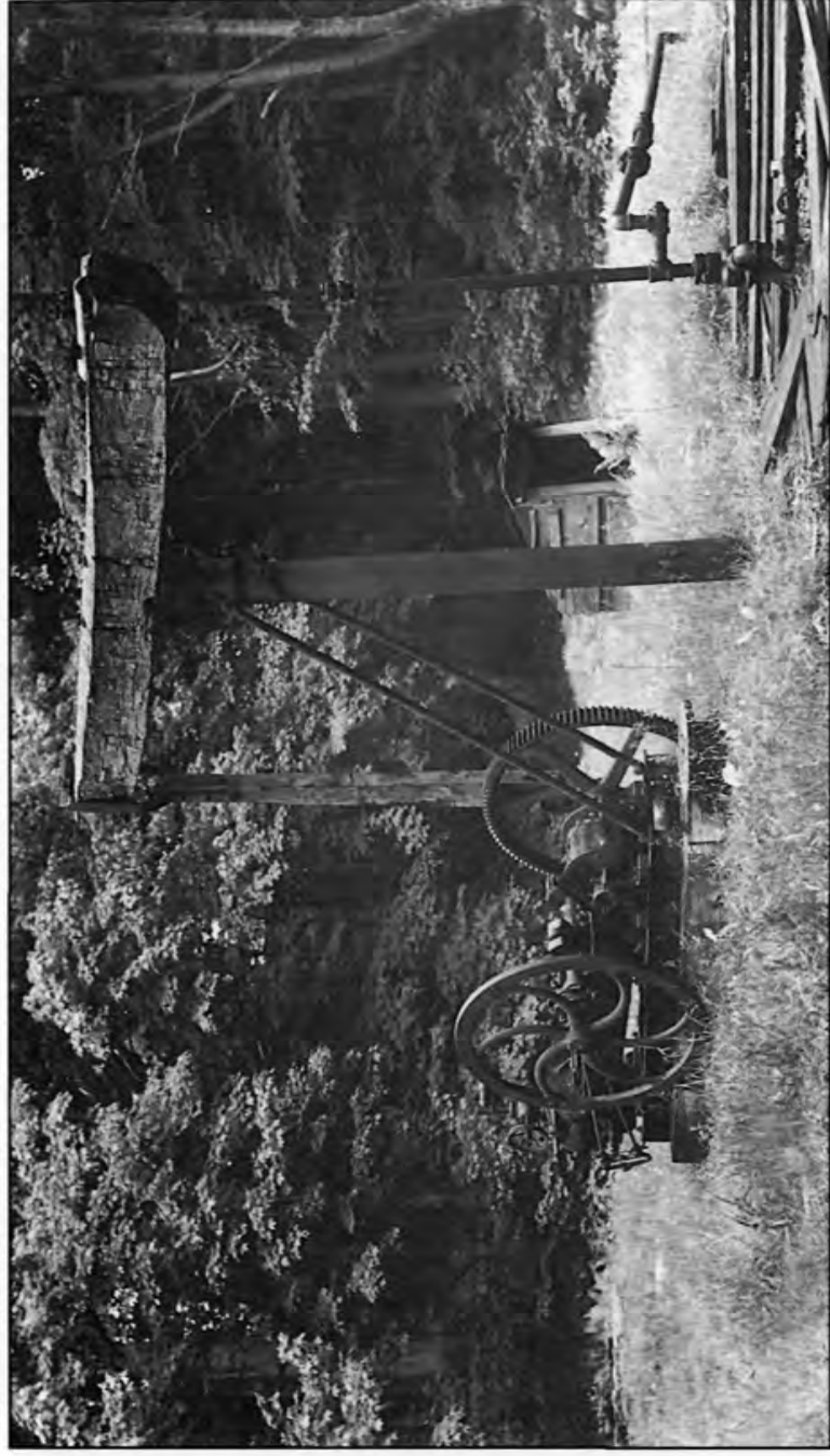
The Forest Service began purchasing much of the surface area of the Middle Field in 1923. The early Allegheny National Forest hosted a well-established producing industry. Pictured here is a Barcroft or "Blaisdell" compressed-air pumping rig, in 1926. Note the modified Farrar & Trefts steam engine. USDA Forest Service
