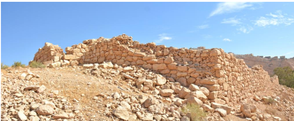
Fig. 5 - The southern wall and the south-western corner of the khan.
