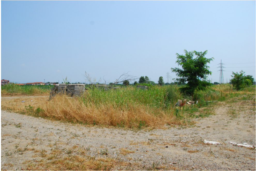
Fig. 3 – Trecella (Pozzuolo) – One can clearly see the state of neglect of an infrastructure only 90% completed by the Italian Rail Network (RFI). The presence of the BreBeMi motorway has reshaped the southern part in order for the foundations of the road to be constructed, while the ramp to the north should be demolished. So far the function of the entire sedimentary area between the support walls of the ramp that have yet to be demolished seems to be uncertain, while the site has been entirely filled with debris from the quarry, becoming a real relict area. Photo by R.G. Rizzo, July 2013.
