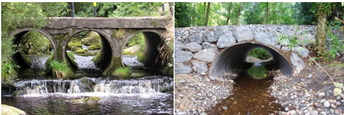
Figure 9. Examples of culverts (photos: Z. Kaczowski (photos: AMBER).
