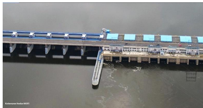
Figure 5. Fishpass on the Włocławek dam – the attraction flow is visible at the entrance of the fishpass (photo: K. Suska, SSIFI, Poland).
