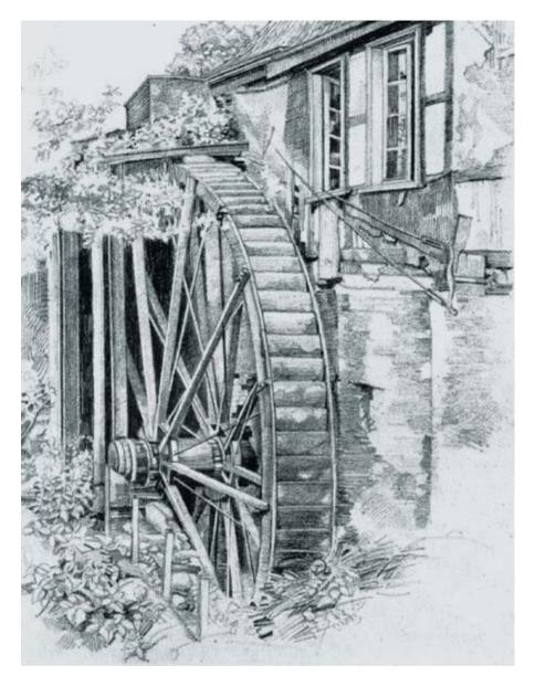
being to derive power from the central axle instead of simply lifting water. The Vitruvian waterwheel drove millstones through gearing—generally at the ratio of 5:1—and were eventually adapted to many differing purposes as the availability of slaves decreased.
