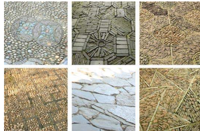
Figure 11. The pavement of different materials and textures in Jiangnan Gardens.
