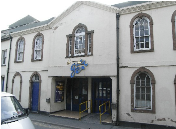
The Grade II listed County/New Regal Hereford – photo taken April 2010
