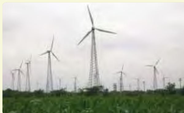
Clean Energy of 12 MW capacity generated by JKM Wind Farm at Coimbatore - a step towards achievement of zero carbon footprint.
