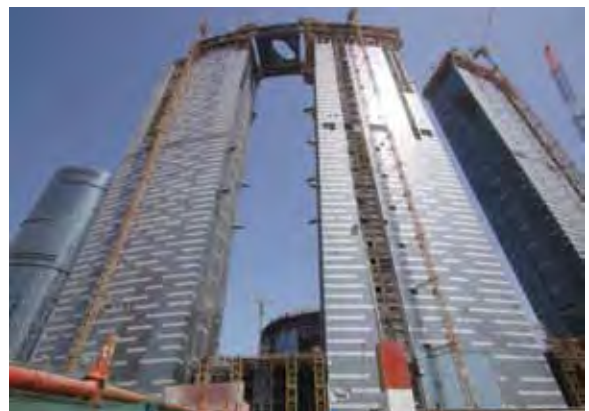
Figure 9. Construction photo series showing installation of skybridge spans.
