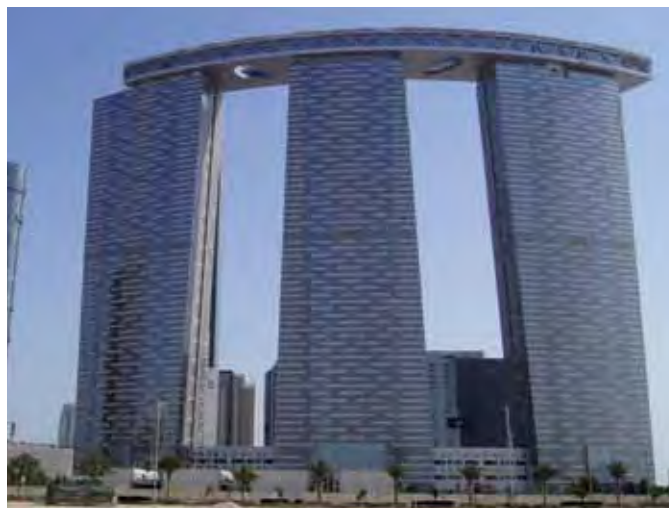
Figure 4. The Gate Towers, tapering shapes.
