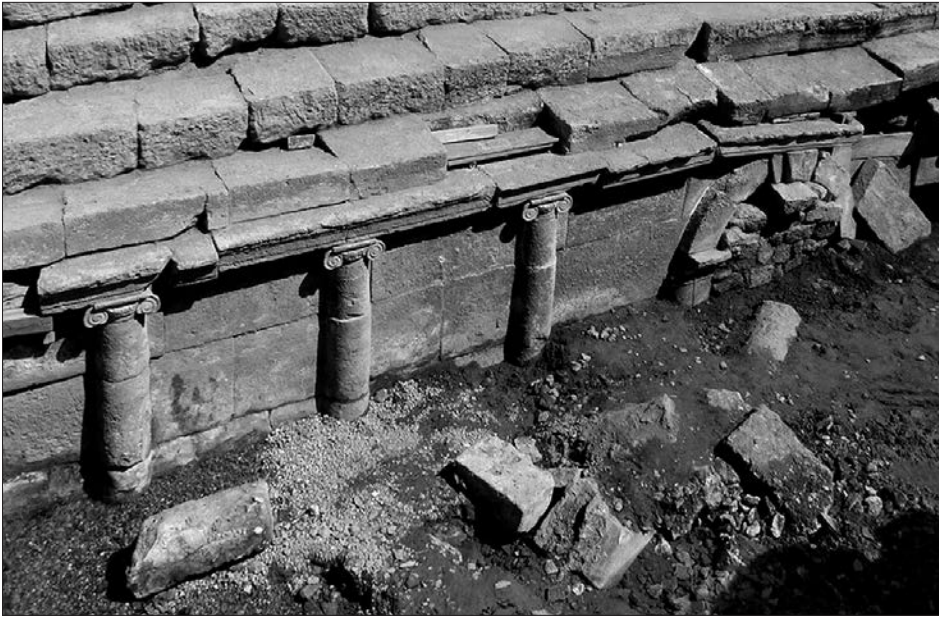
1. - Dumped blocks emerging in front of the Ploutonion's façade during excavation (photo P. Panarelli).
