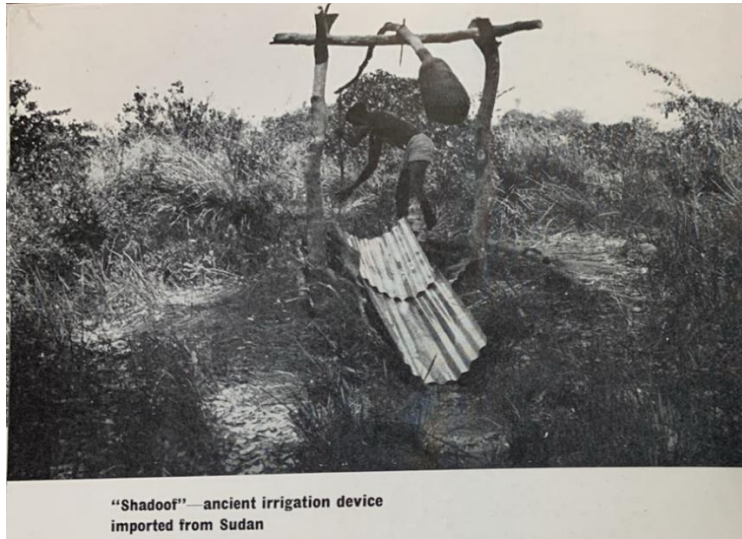
Figure 2-1: A shadoof. (McBow & Ukeje, 1959, p. 10)
