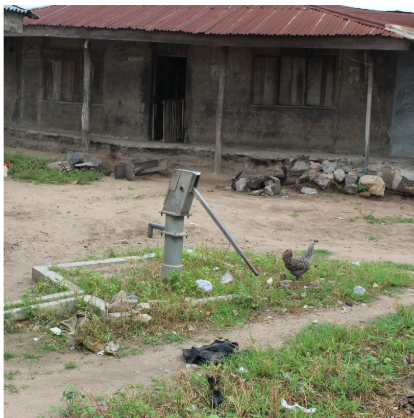
Figure 0-2: An abandoned standpipe waterpoint
