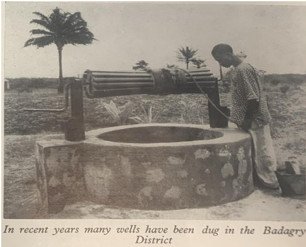
Figure 8-2: The standard ‘traditional’ wells adopted and improvised by the government. Source: (Duckworth, 1952, p. 173)
