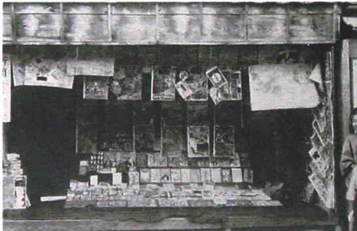
Figure 23: Zauri -style Bookstore, circa 1890. Until the end of the Meiji period, Japanese bookstores were narrow and shallow in order to take advantage of natural lighting. From Hyakunen mae no Nihon (Japan one hundred years ago), page 122.
