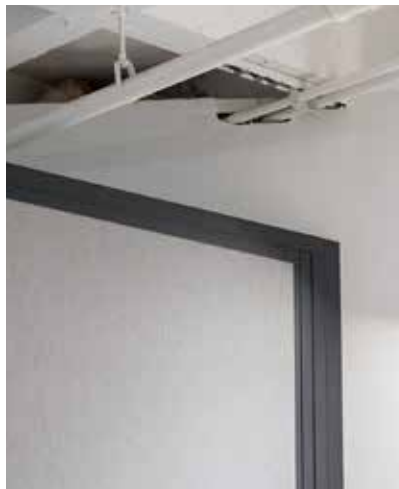
ANGLED WALL START WOOD BLOCKS CAN BE SPECIFIED TO ACCOMMODATE SITE WALL ANGLES OF BETWEEN 3 AND 87 DEGREES (Curved Wall Pictured Above)
