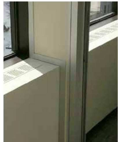
MONOLITHIC INSERT PANELS WITH VINYL OR HPL SURFACES CAN BE CUT ON-SITE TO ACCOMMODATE IRREGULAR WALL CONDITIONS, USING TRADITIONAL CROWN FOR TRIM AROUND THE CUT EDGES
