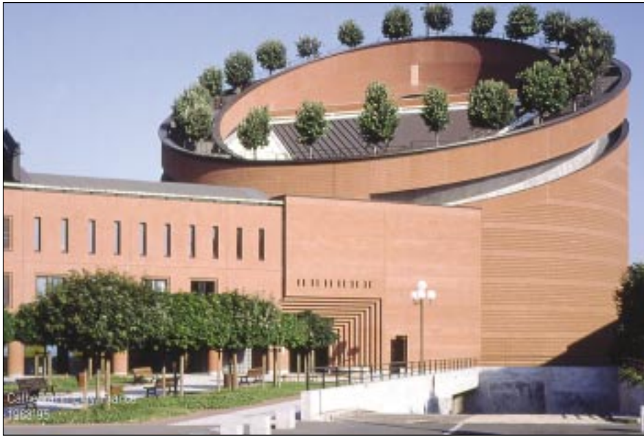
The Cathedral of the Resurrection (1988–95) at Evry, France, is located just south of Paris. A truncated cylinder, it is made of reinforced concrete clad inside and out with some 800,000 red bricks from Toulouse, an homage to the artisans of the medieval French cathedrals and the local masonry tradition. A ring of lime trees, like a green halo, marks a walkway along the upper reaches of the church.
