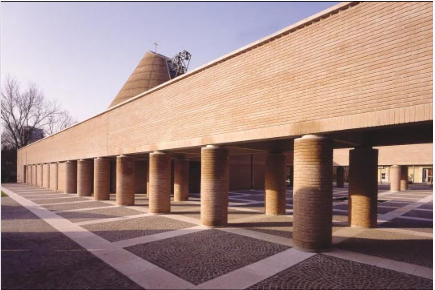
The Parish Church of the Blessed Odorico (1987–92) in Pordenone, Italy, the plan of which consists of a rectangular, colonnaded courtyard that frames a central conical bell tower, the terminus of which is cut on a diagonal and completed with a slanting circular skylight, iron belfry, and cross.
