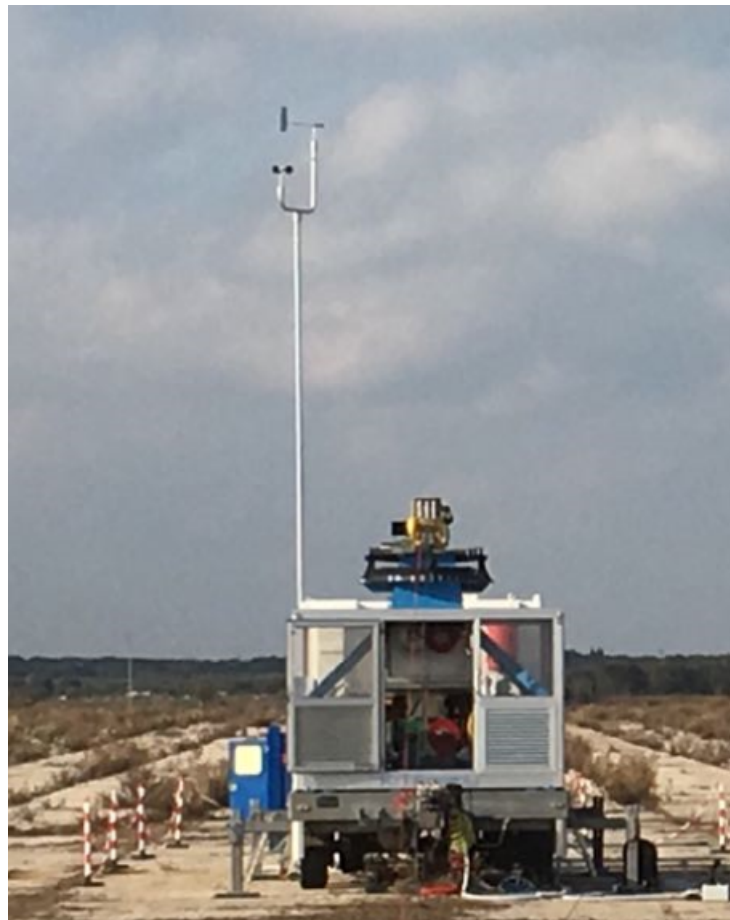
Figure 4.9: Wind station installed and working on the field.
