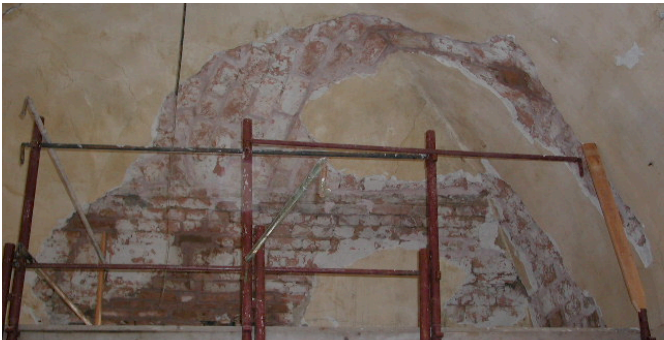
Figure 6. Detail of a vault in palazzo Pallavicino Ariguzzi.
