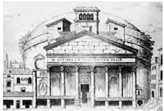
Figure 54. The Pantheon in the early 17th century. Two columns and three capitals of the portico are missing. The pediment is broken; a bell tower marks its use as a church
