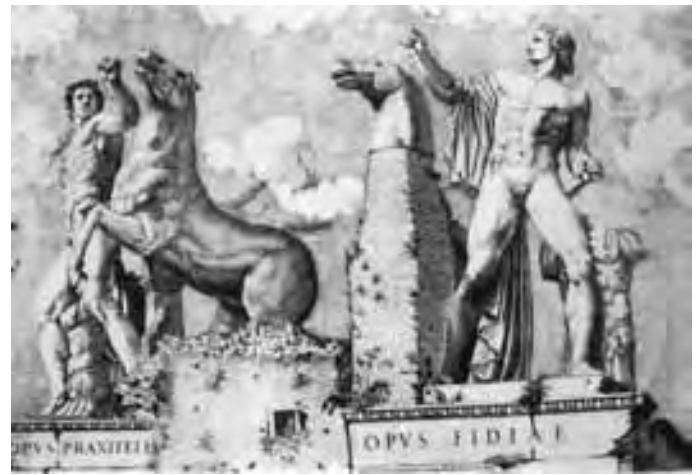
Figure 21, An example of 14th-century restoration of a public monument, the ‘Dioscuri’, with the support of brick walls (Rome, c. 1550)
