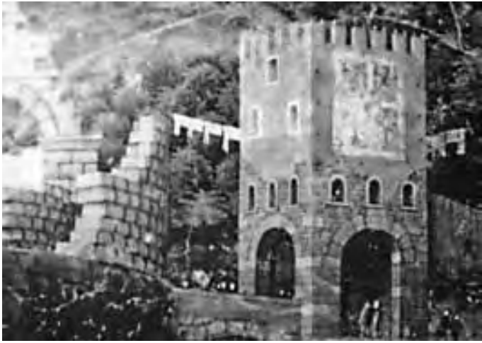
Figure 13. Detail of a 15th-century painting by Andrea Mantegna, showing restoration of a tower
