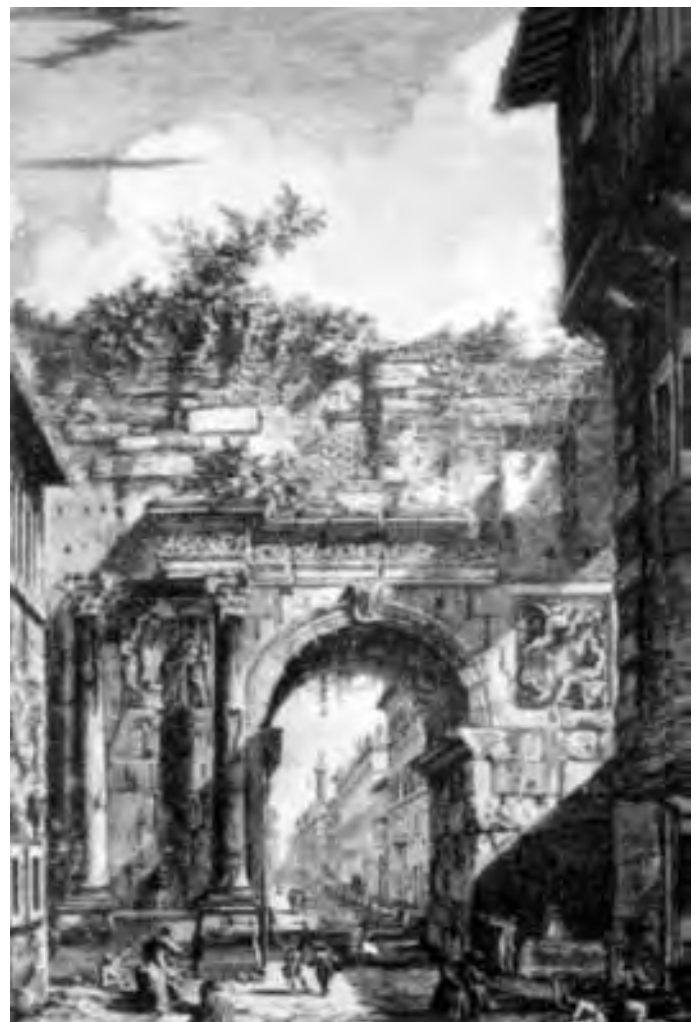
Figure 52. Arco di Portogallo in Via Flaminia, today Via del Corso, Rome, demolished because considered obstacle to traffic
