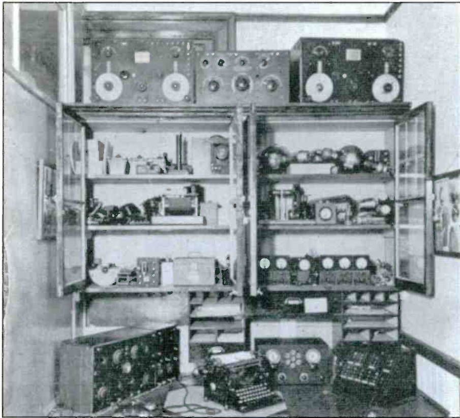
Commercial Receiving Room and testing apparatus.
