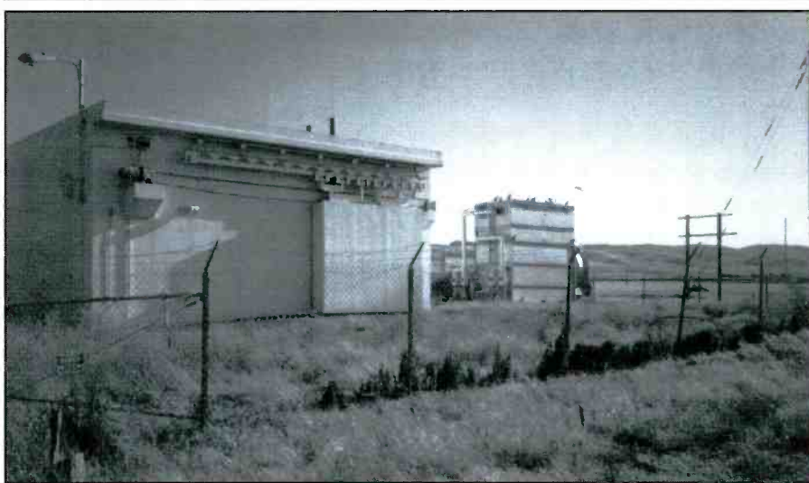
View of building with surrounding fence.
